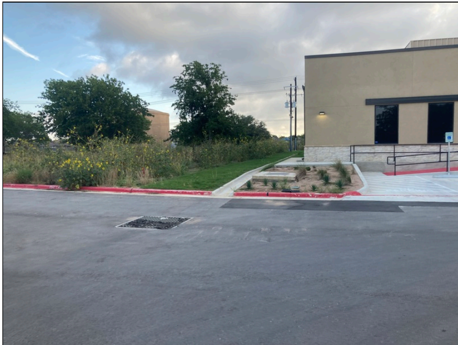
12 - Northwest property corner facing north
