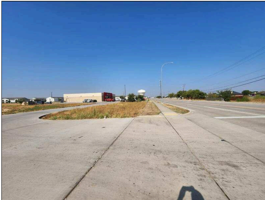
4 - North boundary looking west
