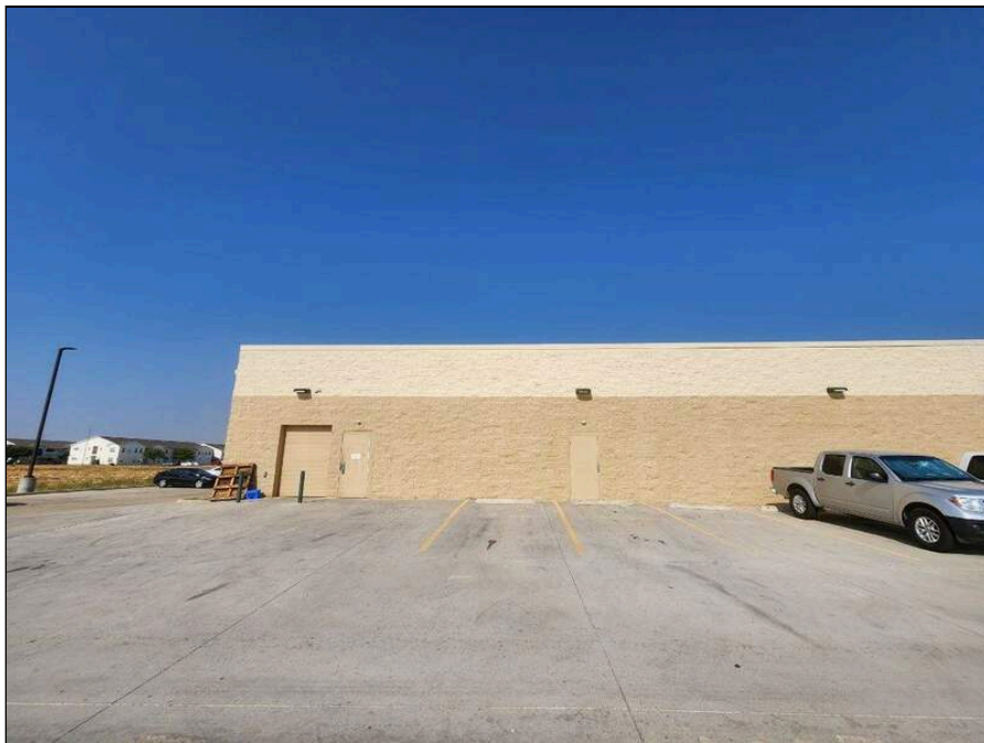
14 - Adjoining property to the west
