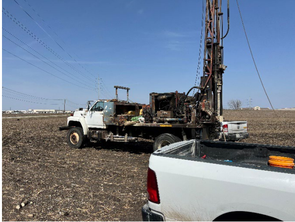
Boring B-01 Facing North
