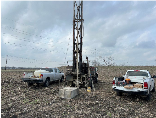
Boring B-05 Facing North
