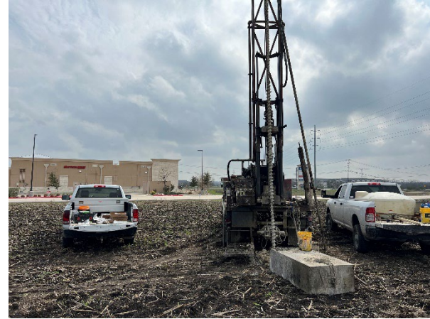
Boring B-02 Facing South
