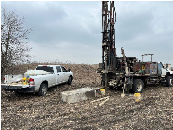
Boring B-07 Facing Southeast
