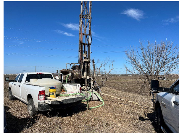
Boring B-08 Facing West
