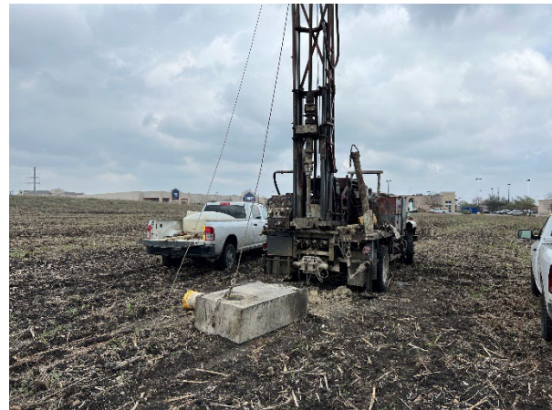
Boring B-15 Facing Northeast
