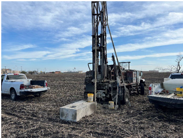
Boring B-13 Facing South
