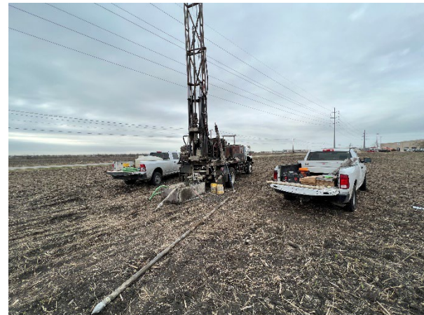
Boring B-04 Facing North
