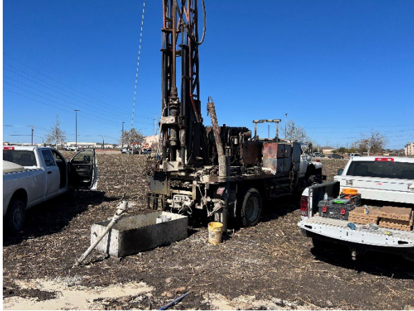
Boring B-09 Facing North
