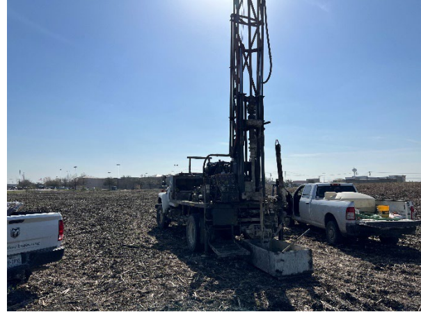
Boring B-11 Facing South
