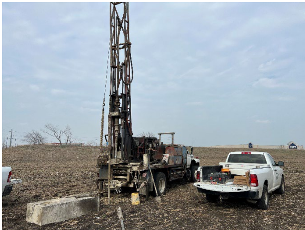
Boring B-03 Facing Northeast
