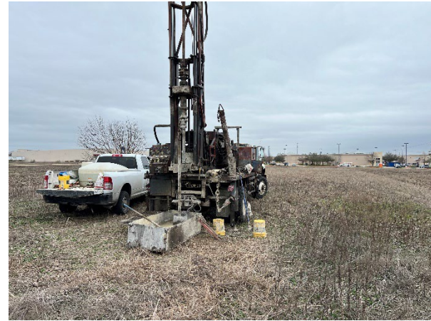
Boring B-06 Facing East
